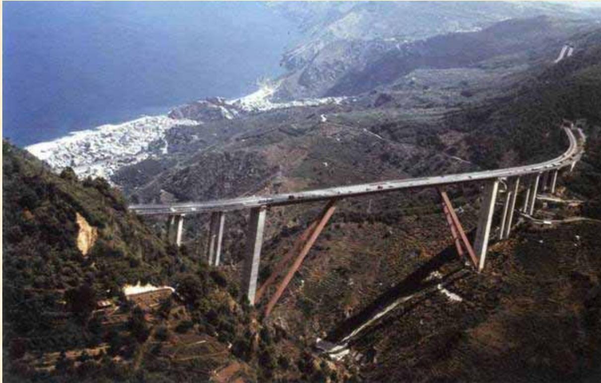
Sfalassa ravine viaduct in Italy, 376 metres span between pier centre lines (1973), S. Zorzi, L. Lonardo and S. Procaccia. The largest frame bridge in the world.
