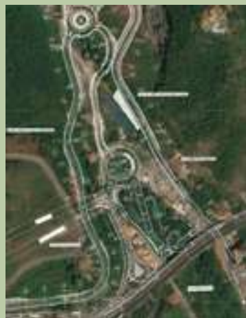
Completion of the Salerno backport road system, the Porta Ovest lot, section I, 2022
