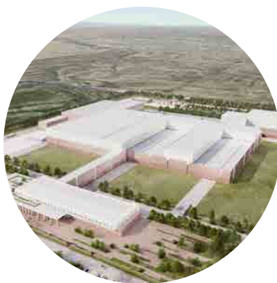
POLITECNICA PMI INDUSTRIAL FACTORY, DENVER, USA
