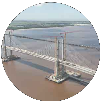
POLITECNICA NEW DEMERARA RIVER BRIDGE, GUYANA
