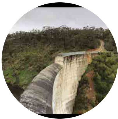
SPERI CONSULTANCY AND FINITE ELEMENT ANALYSIS FOR THE STURT RIVER DAM RAISING PROJECT IN ADELAIDE, AUSTRALIA
