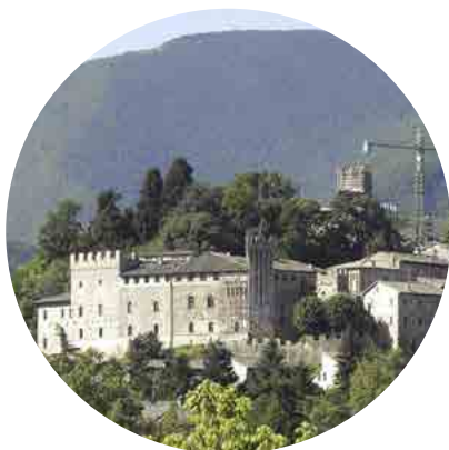
FIMA RESTORATION OF PALLOTTA CASTLE, ITALY
