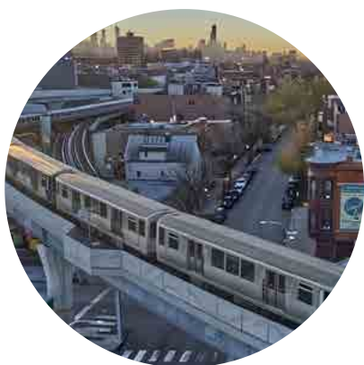
RINA PROGRAM MANAGEMENT OFFICE, CHICAGO METRO NETWORK, USA
