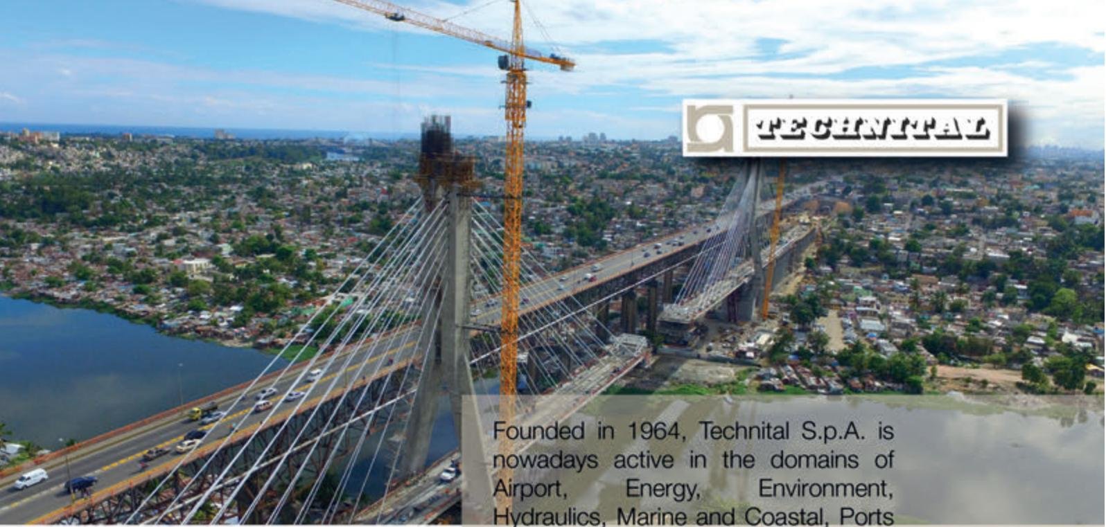
An aerial photograph of a large cable-stayed bridge under construction. The bridge spans a wide river. Several tall concrete pylons are visible, with numerous stay cables fanning out to support the bridge deck. A large yellow tower crane stands prominently on the bridge deck. The surrounding area is densely populated with residential buildings and greenery.
