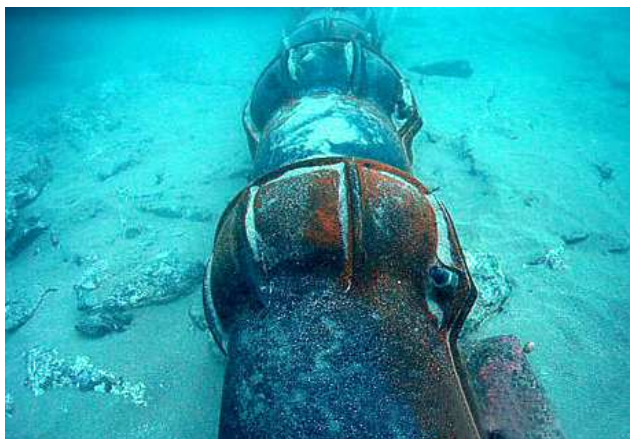
Cable laid on the seabed and protected by Cast Iron Shells Installation
