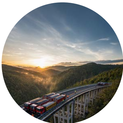
MASERA TECCIO VIADUCT - STATIC LOAD TEST, ITALY
