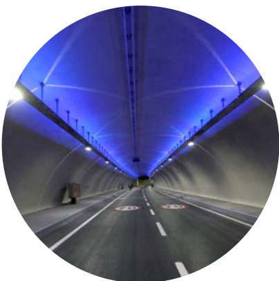
FS ENGINEERING EURASIA TUNNEL, TURKEY
