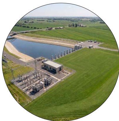
TECHNITAL WATER PUMPING STATION, CAVALIERA, FERRARA, ITALY
