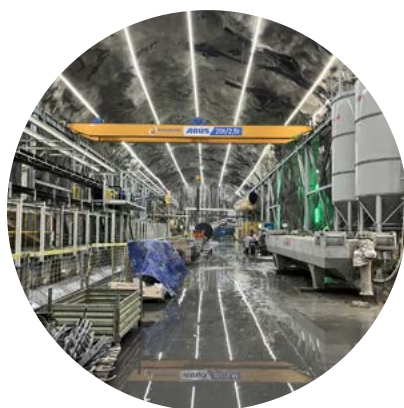
SYSTRA SPA RENTVANNSTUNNEL, OSLO, NORWAY
