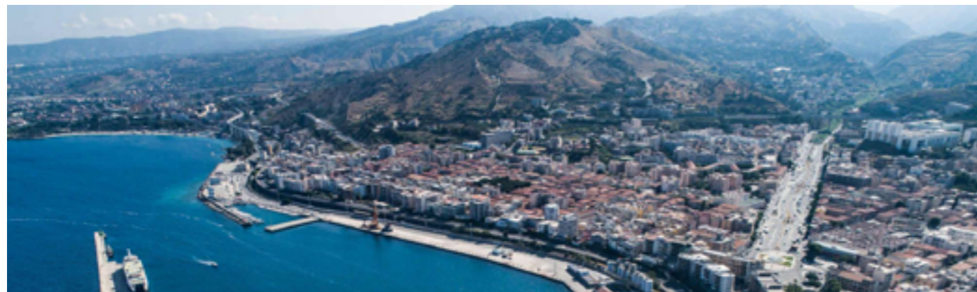
The route will extend between the second and third rows of warehouses in the Old Port. The project includes a connection to the center of Trieste in the south and to the Bovedo parking lot in the north. The Old Port and the city of Trieste as a whole have always had a European and international character, and therefore the project relates to this supranational dimension.
