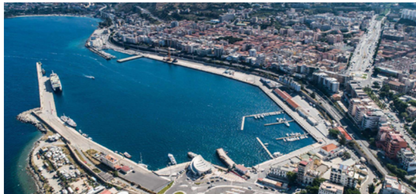
The project enhances the functions of the port's outer basin through the construction of a new passenger terminal for cruises and the inner basin with the redevelopment of the old quay and the repurposing of existing buildings for recreational boating. This intervention enhances the interaction between the port and the city, improving accessibility, services, and tourist appeal.
